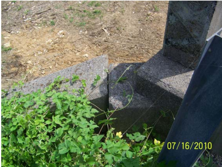
Headwall Separation at Culvert
