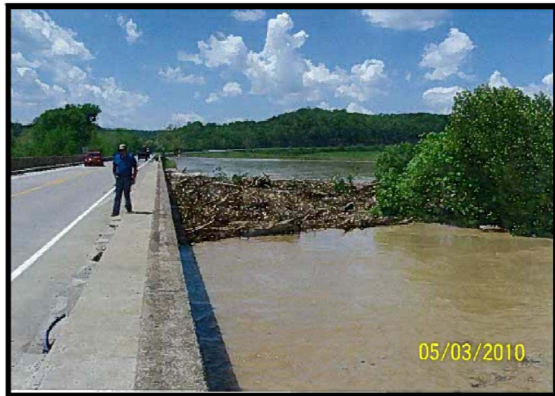
Figure 11: Highwater and Drift Accumulation at the Bridge over Beech Fork
