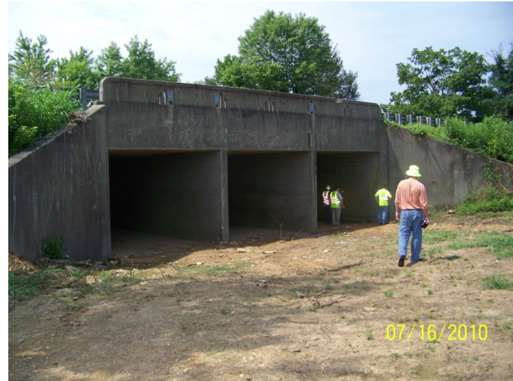
Three Span Culvert (Beech Fork Overflow)
