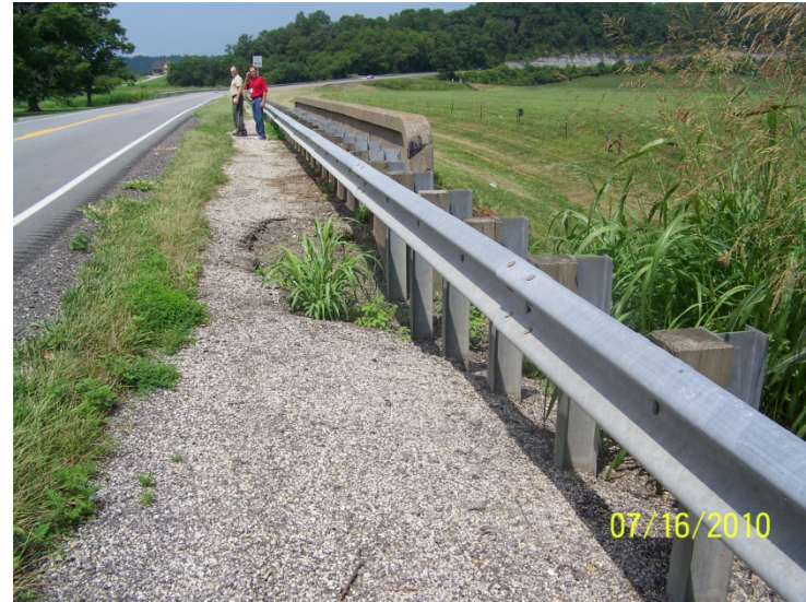
Headwall at Culvert (Roadway Drainage Problems)
